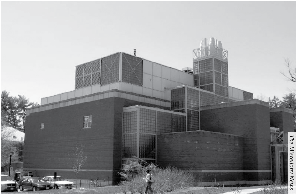
The improvement of Vassar’s science facilities will be concluded in 2017 with the demolition of Mudd Chemistry Building, pictured above. The Chemistry Department will move to the new bridge building.
